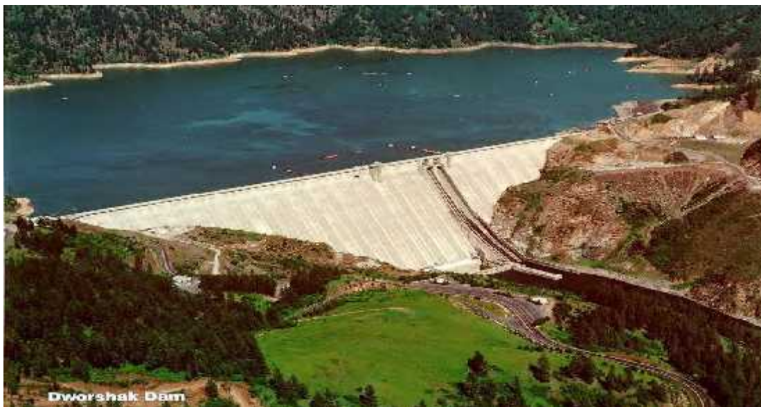
Fig 10.2 Gravity dam - Dworshak Dam
