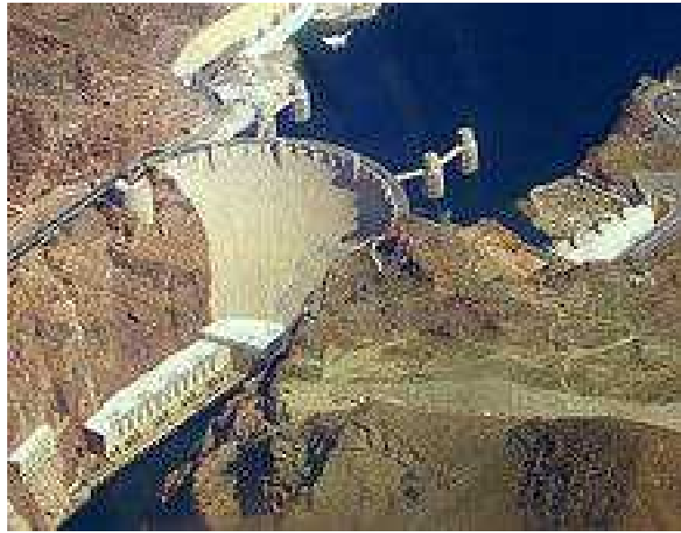
Fig. 10.1: Arch-Gravity Hoover Dam
