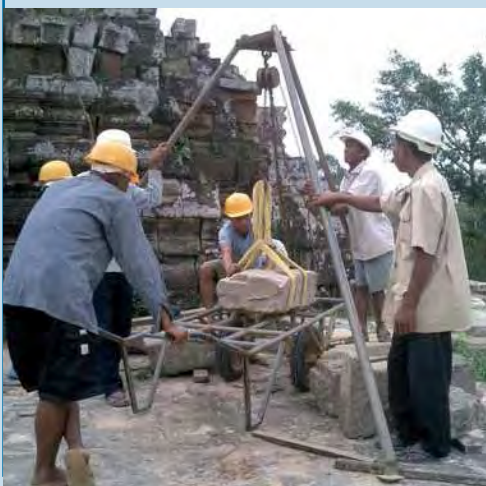
Moving heavy stone materials by using local, available methods
